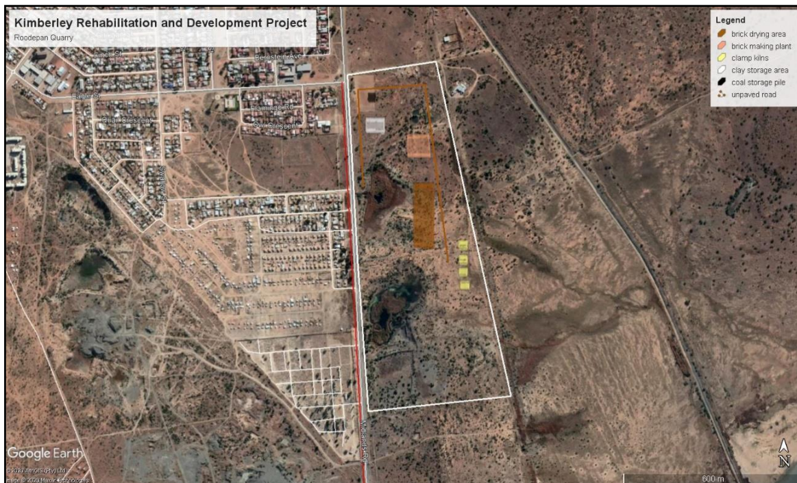
Figure 12-1: Assumed site layout of activities at Roodepan Quarry and Clay Brick facility
