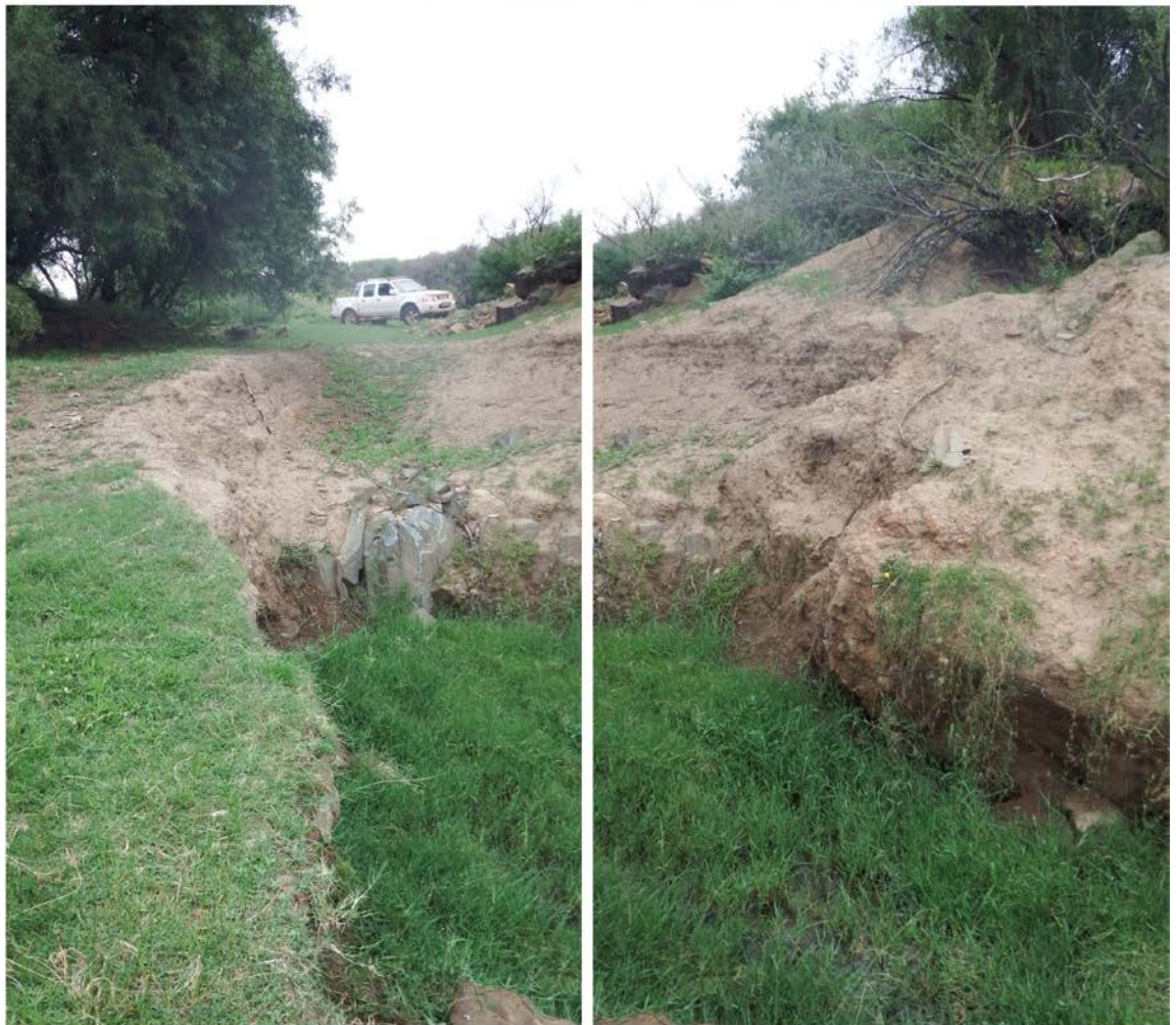
Figure 11. Geologically recent alluvium and sandy overbank deposits exposed along the banks of the Vaal River.
