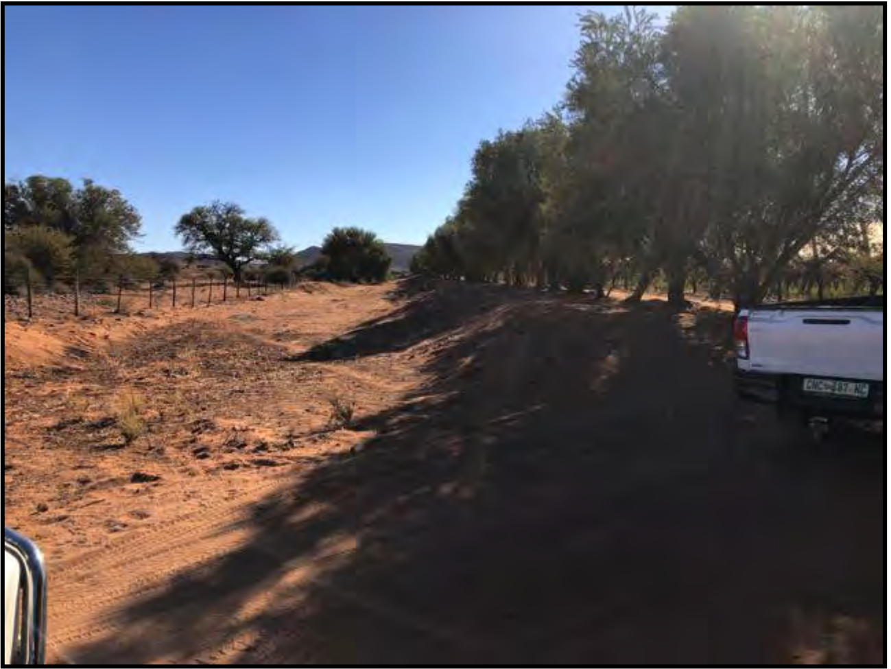
Stormwater drainage berms
