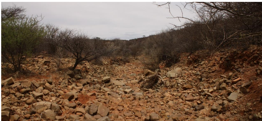
Figure 29: View of one of the drainage lines within the interior of the rocky, uneven central portion. A main channel is still prominent although riparian vegetation is largely absent.
