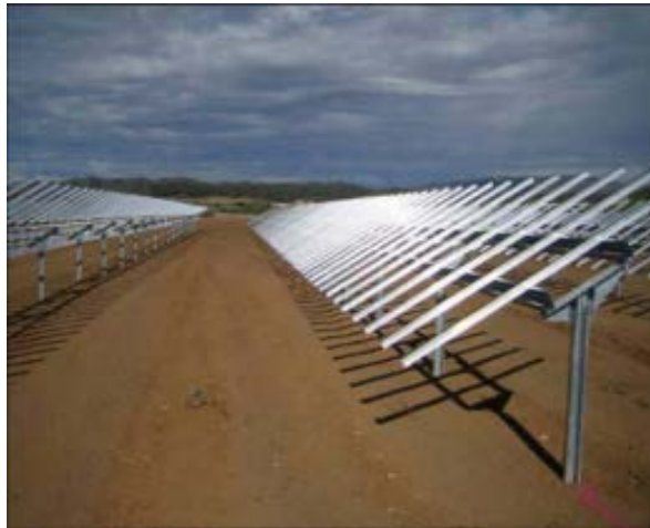
Figure 6: Completed PV Panel Mounting
