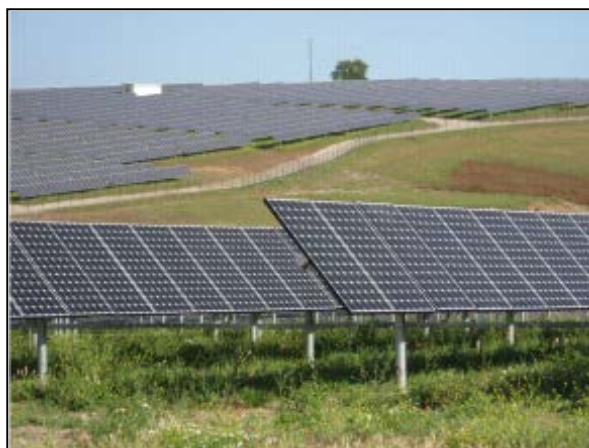
Figure 7: Completed PV Panel Structures
