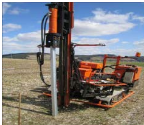
Figure 5: PV Panel Foundation Construction
