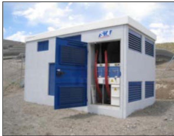
Figure 8: PV Panel Inverters
