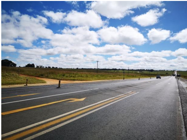
Image 1 - N4 east-facing with Access Road 1 on the left
