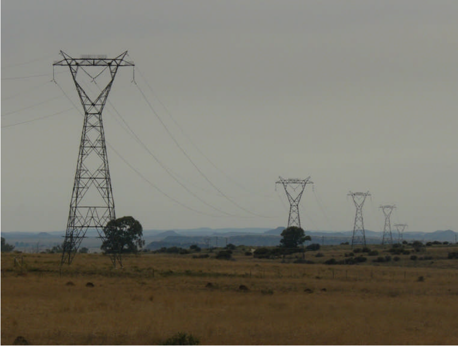
Plate 3 The visual impact of transmission power lines on a flat landscape.
