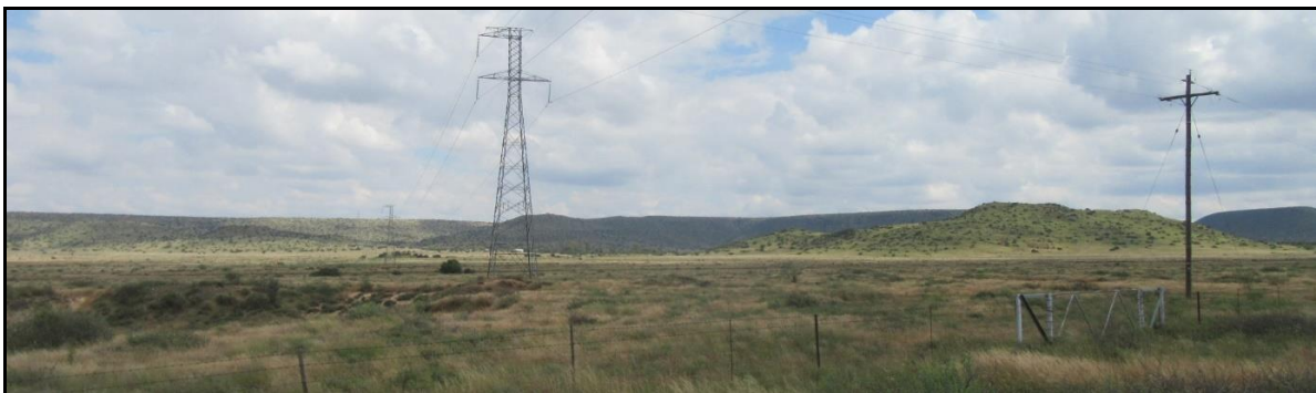
Photograph 3.4: Transmission line on Ruspoort
