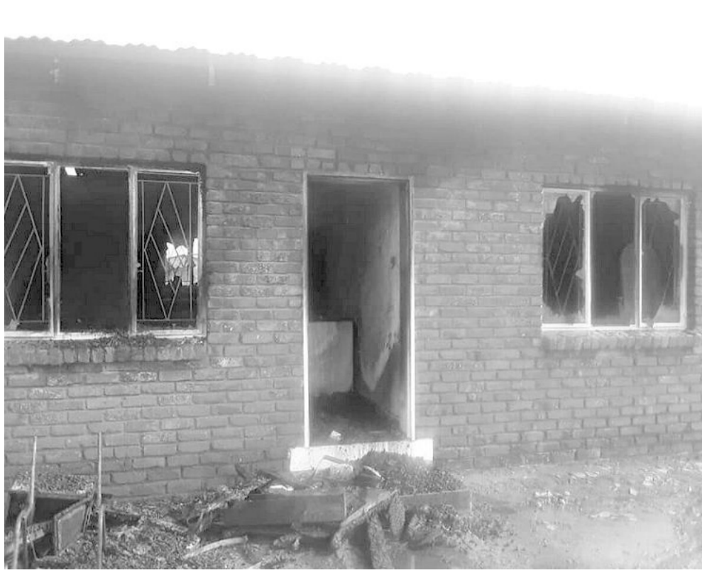
A house fire was extinguished in Mossie street on Sunday.
