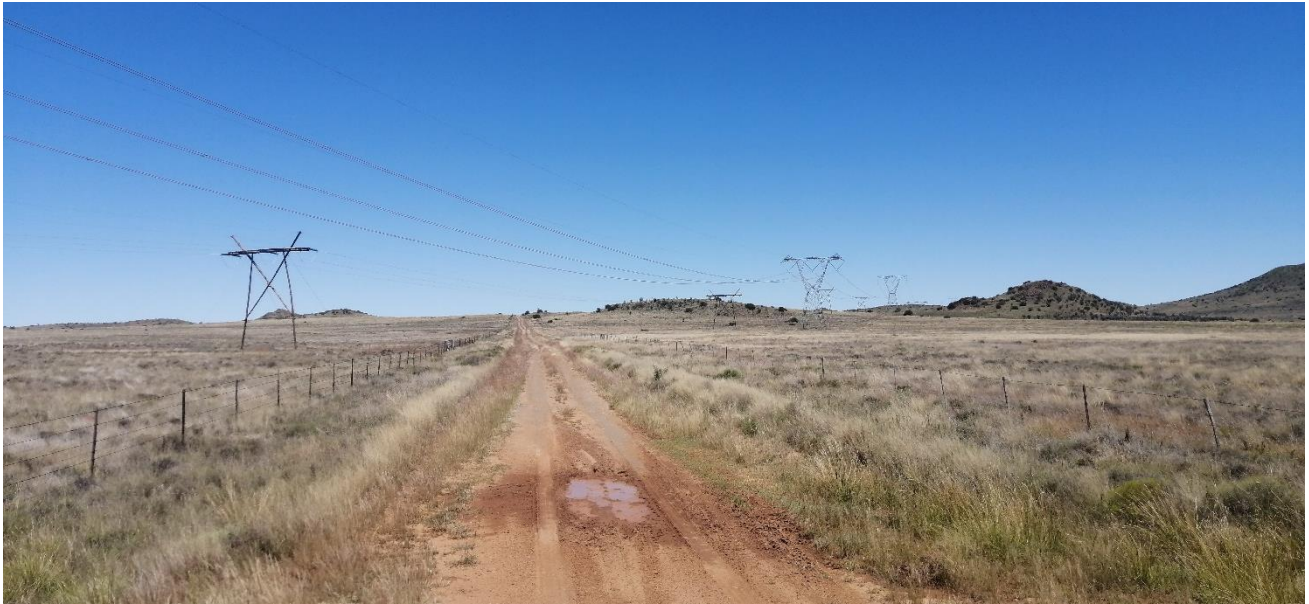
Figure 13: An example of a secondary road traversing the study area
