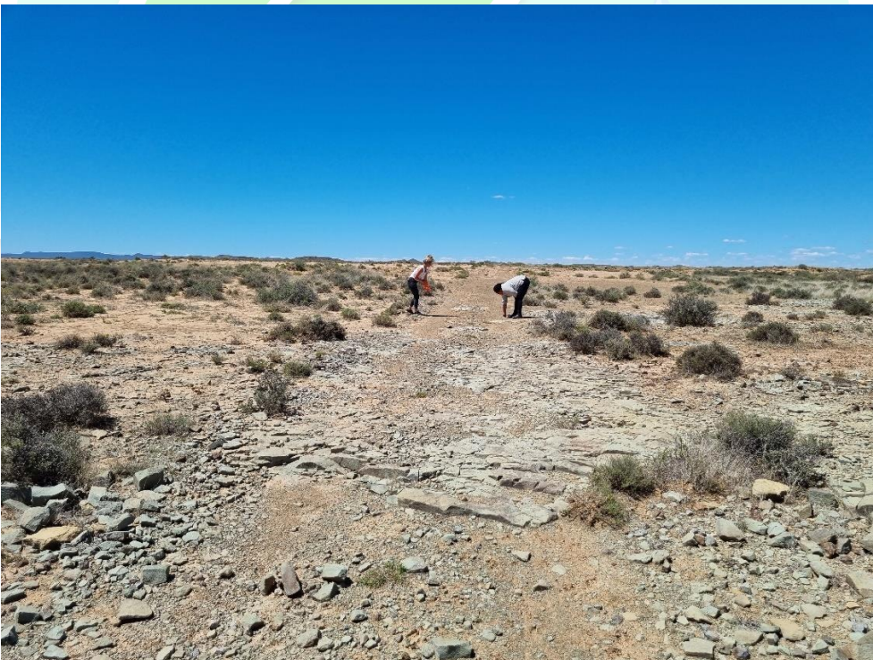
Photo 13. Private road crossing/farm track over the Brak River and flood plain.
