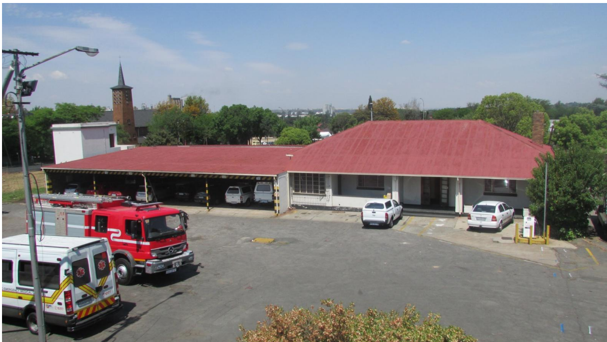
Figure 10: View of other structures in the area proposed for development.
