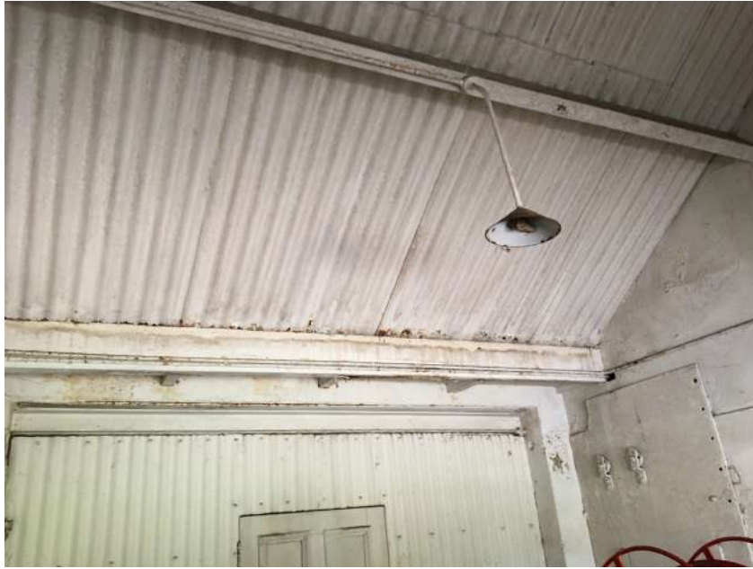
Fig. 5 – exposed roof in the existing “garage” area
