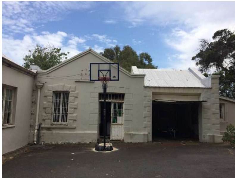
Fig. 2 - Existing building front façade, with garage alteration
