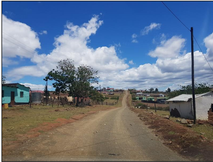
Figure 3-3: View of an existing village road to be upgraded as temporary road in Ndabakazi.
