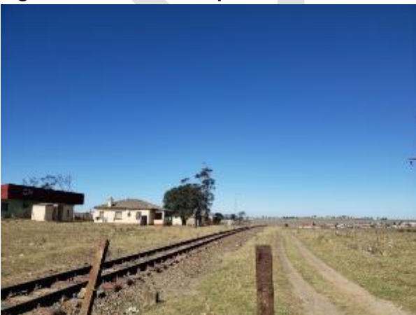
Figure 2-12: View of Photo 1
