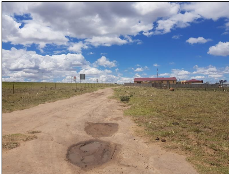
Figure 3-16: View of a dirt road along the N2 (left) to be upgraded as temporary road. Ndabakazi is visible in the distance.
