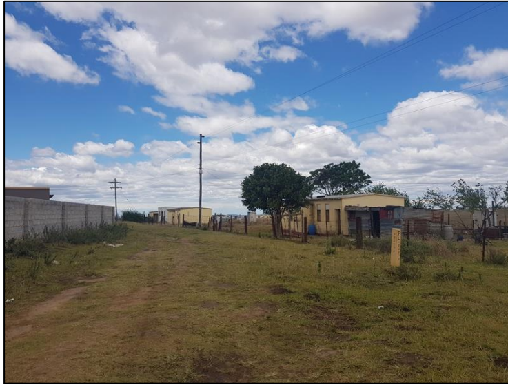
Figure 3-11: View of an open erf north of Ndabakazi where a temporary road will be constructed.
