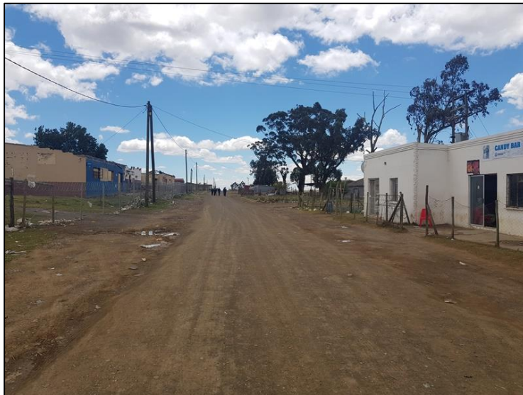
Figure 3-9: View of an existing village road through an industrial zone of Ndabakazi, be upgraded as temporary road.
