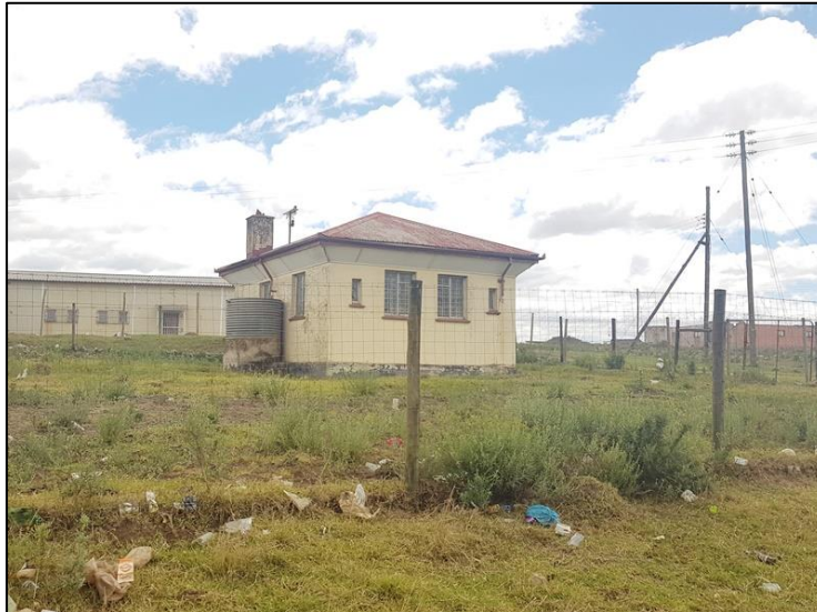
Figure 5-2: The Historical Period building noted at Site Exigo-NIU-HP01.
