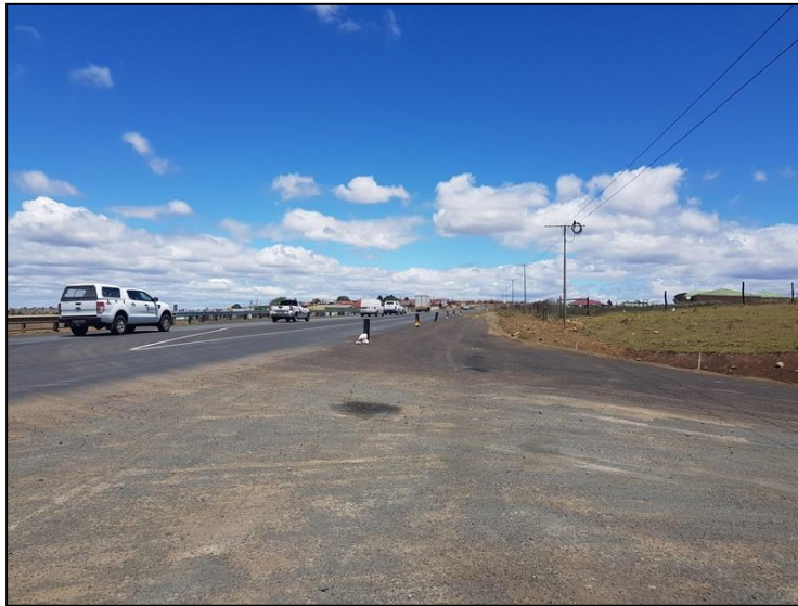
Figure 3-17: View of the N2 to be upgraded at Ndabakazi.
