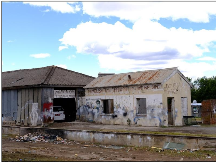
Figure 5-3: View of the Historical Period Ndabakazi station building at Site Exigo-NIU-HP02.
