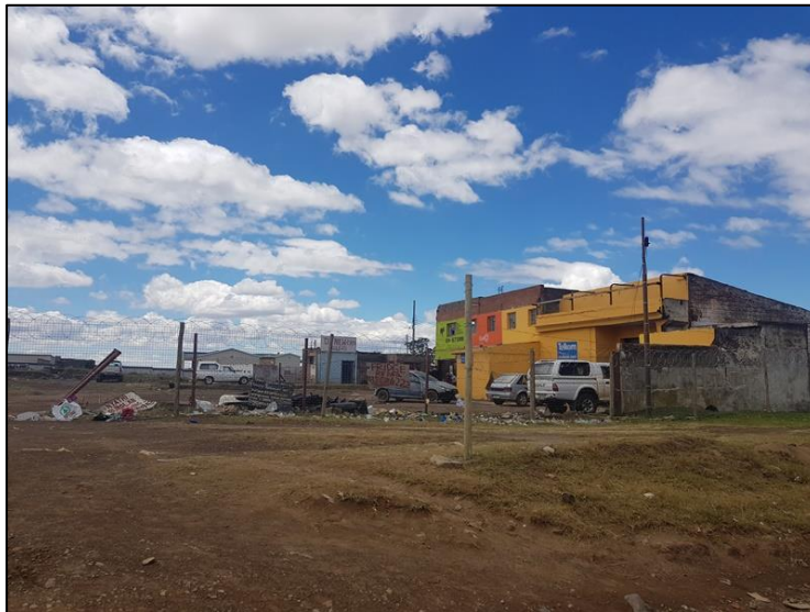
Figure 3-15: View of a small industrial zone at the current Ndabakazi N2 intersection, to be upgraded.
