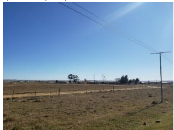
Figure 2-13: View of Photo 2
