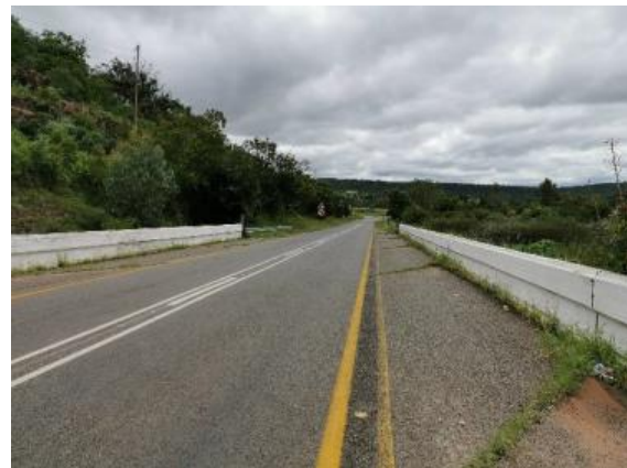
Figure 10: Existing bridges to be replaced
