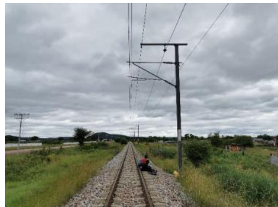
Figure 12: Railway line parallel to R101 at km 1.0
