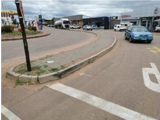
Figure 7: Pedestrian walkway at the start of the project
