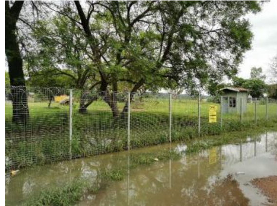
Figure 8: Road section with poor drainage
