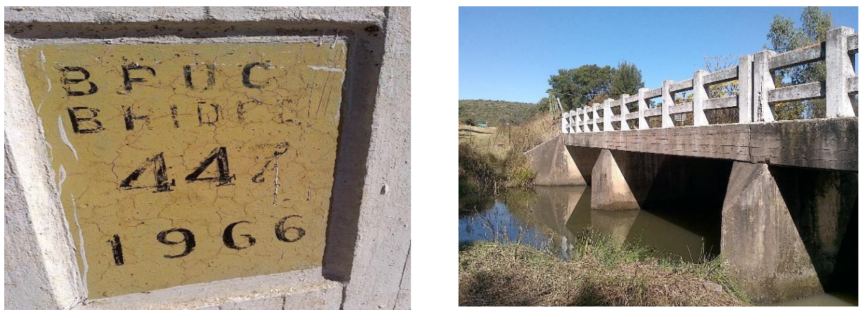
Figure 29: Groot Nyl River Bridge (HCAC, 2021)
