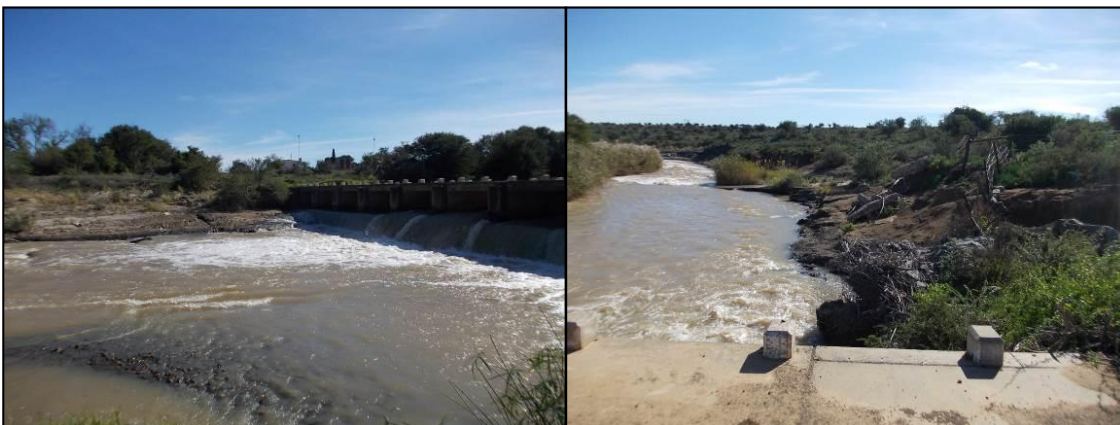
Figure 16: Turbulent flow, erosion and incision associated with sites 9 (left) and 10 (right).
