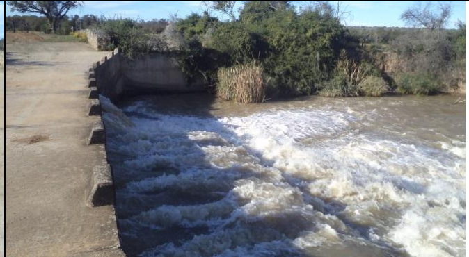
Figure 27: Downstream view of the Site SM1 also showing bridge infrastructure.
