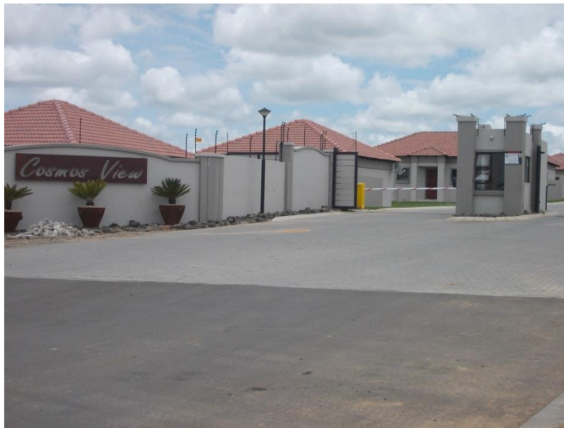
Figure 20: Occupied Cosmos View Complex in Terra Nova
