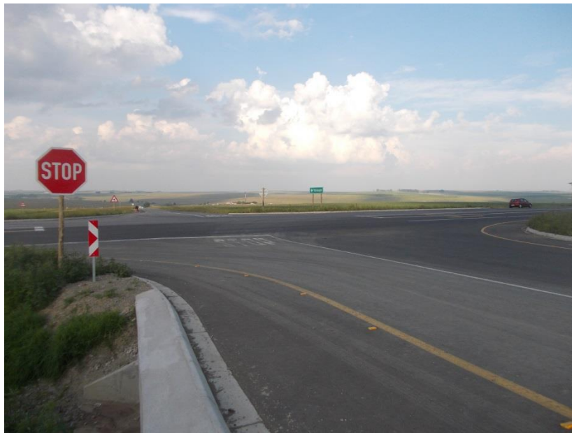
Figure 21: N 17 intersection at Trichardtsfontein Extension 8
