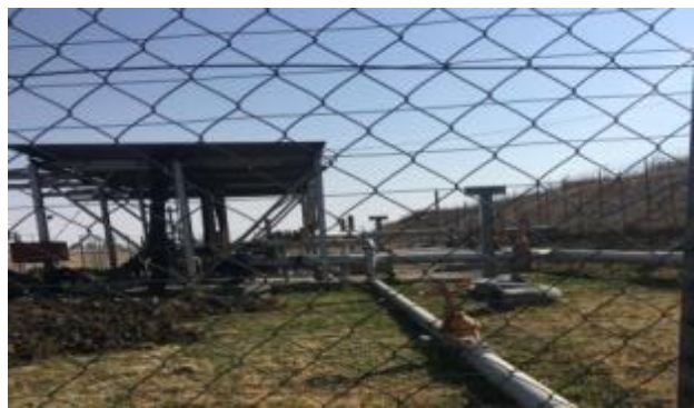
Photograph 7-4: Existing Pump Station
