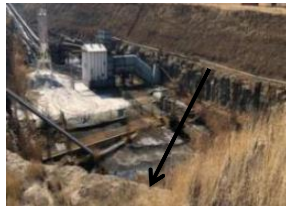
Photograph 7-9: Sump Located at Incline
