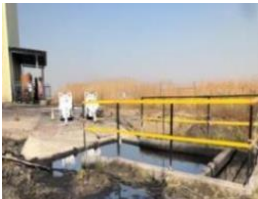
Photograph 7-8: Sump Located at Workshop
