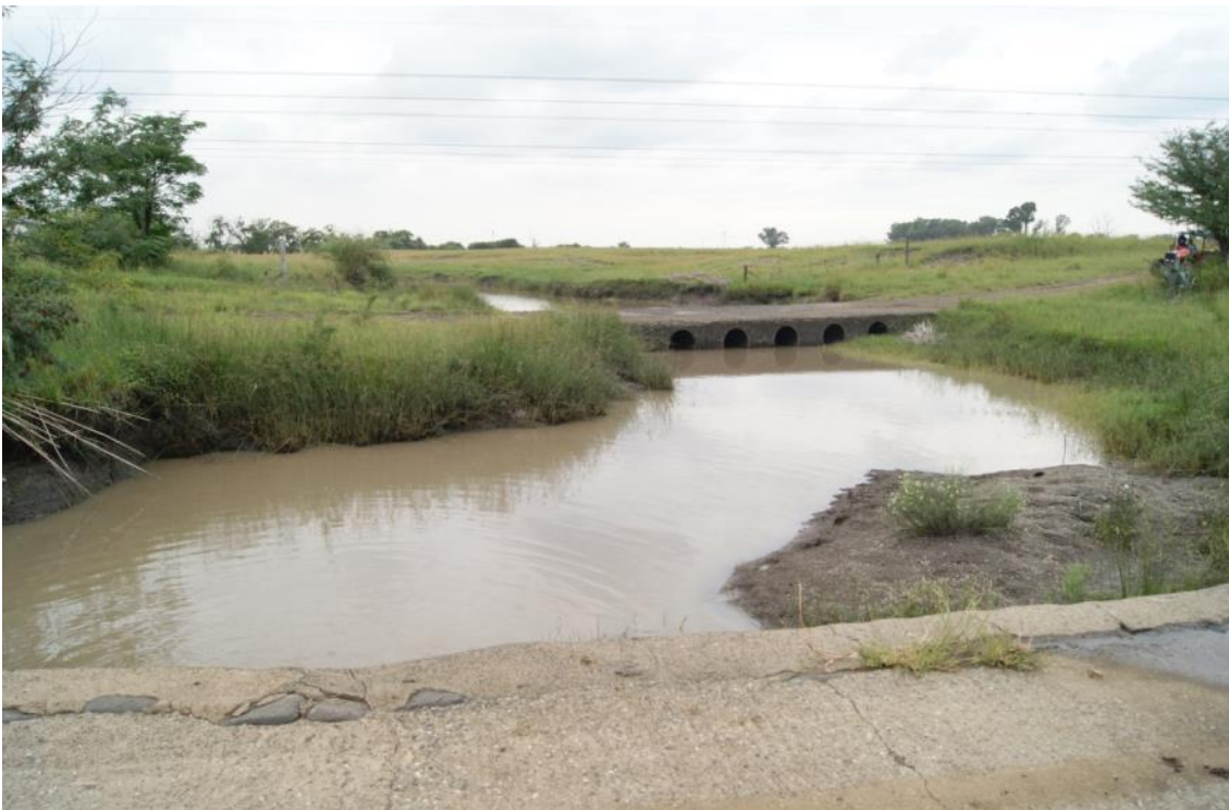
Site KR2 – Downstream site along the Kromelmboogspruit
