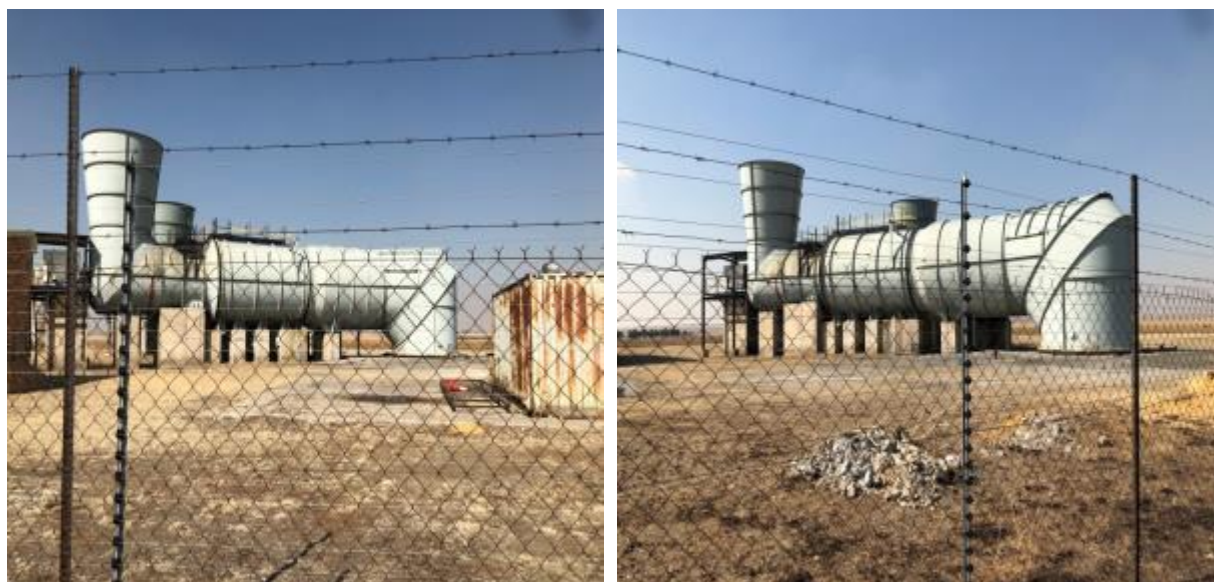
Figure 5-6: Kleinvlei ventilation shaft
