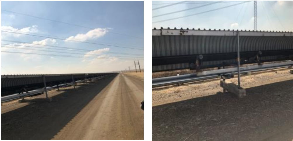
Figure 5-7: Conveyor Belt transporting coal from Mooikraal to 3 Shaft
