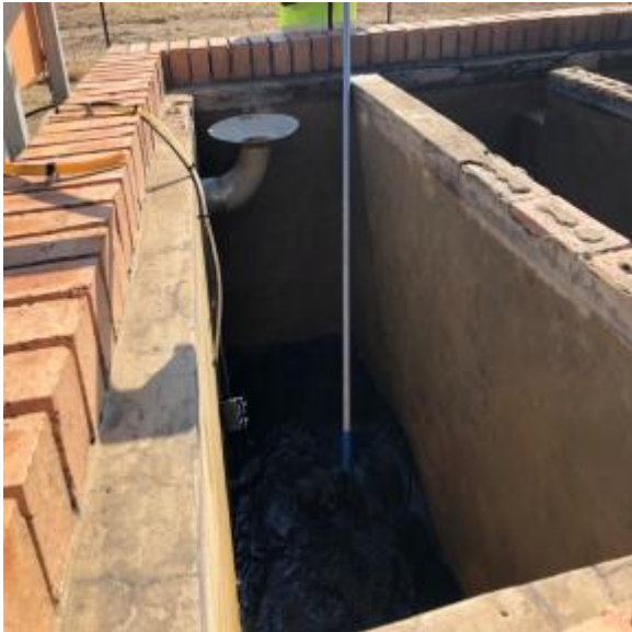
Figure 5-9: Chlorine tank
