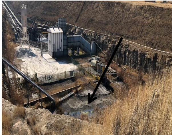
Figure 5-17: Sump located at incline shaft
