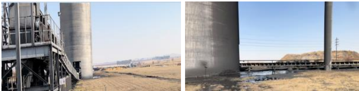
Figure 5-3: Incline, Silo and Conveyor Belt Area
