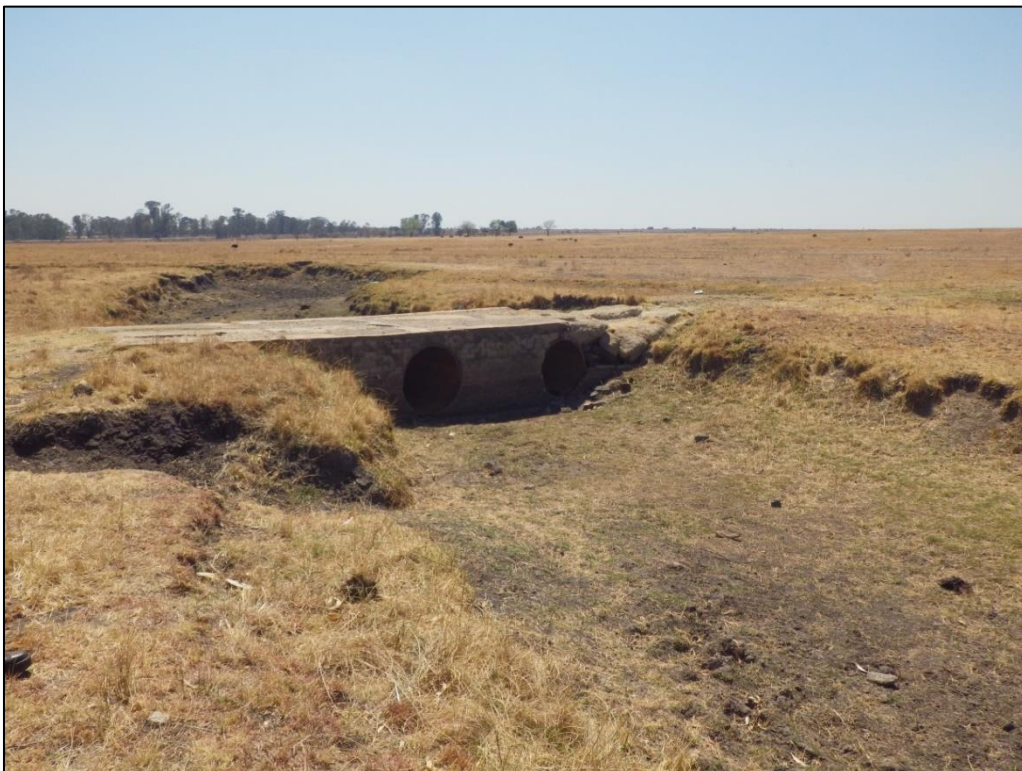
Figure 8-4: The presence of Impoundments such as Weirs and Road Crossings
