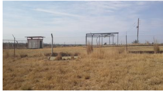
Figure 11-36: Example of a booster pump station located on the existing pipeline route
