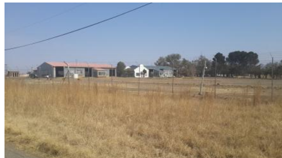
Figure 11-32: One two buildings in the project area. The pipeline will be placed in the servitude (cf. Figure 11-33)
