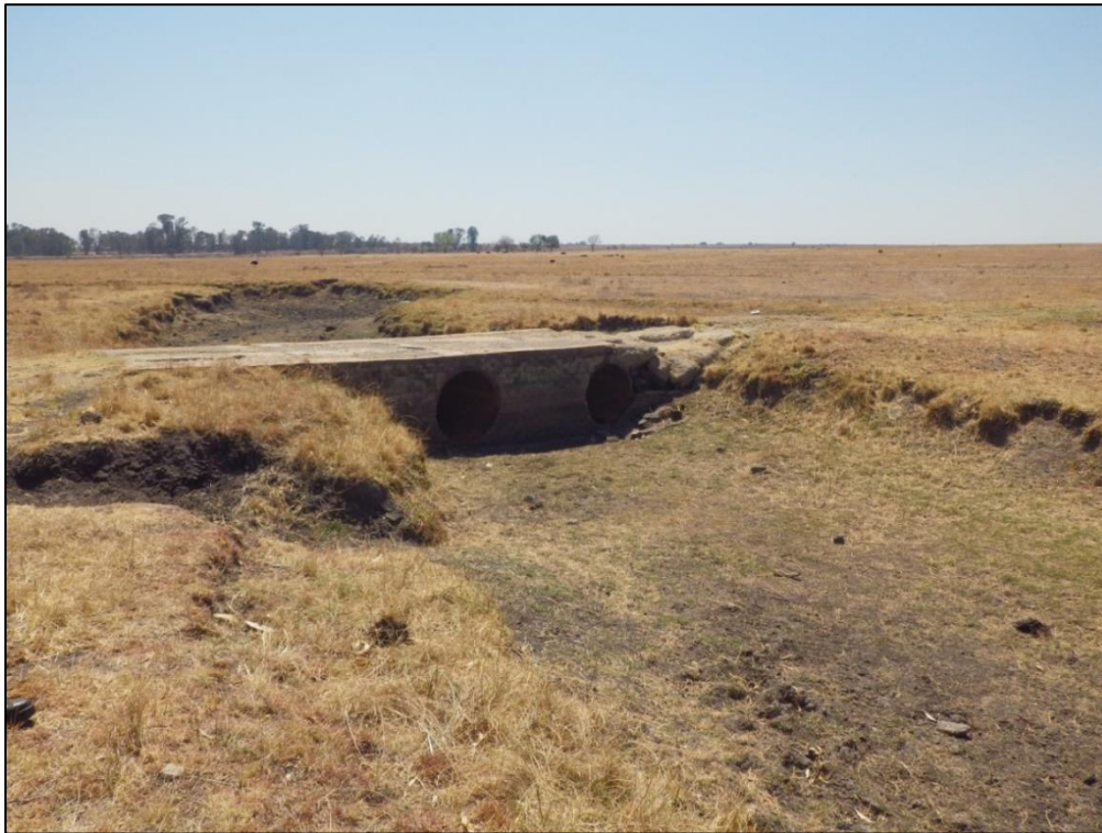
Figure 11-3: The presence of impoundments such as weirs and road crossings
