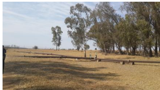
Figure 11-34: General view of existing ash pipeline
