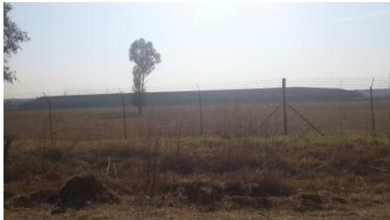
Figure 11-31: Rehabilitated area between fence and tailings
