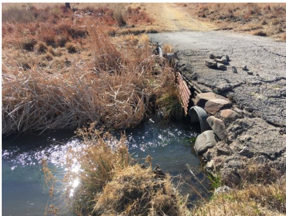
Photograph 20: Local of Leeuspruit (SRD9)
