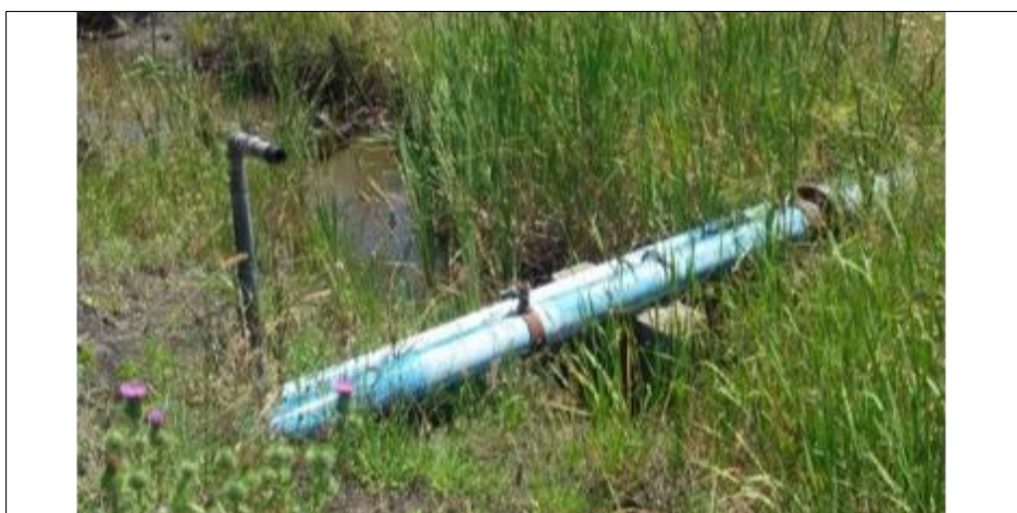
Photograph 5-7: Water pipeline to be decommissioned
