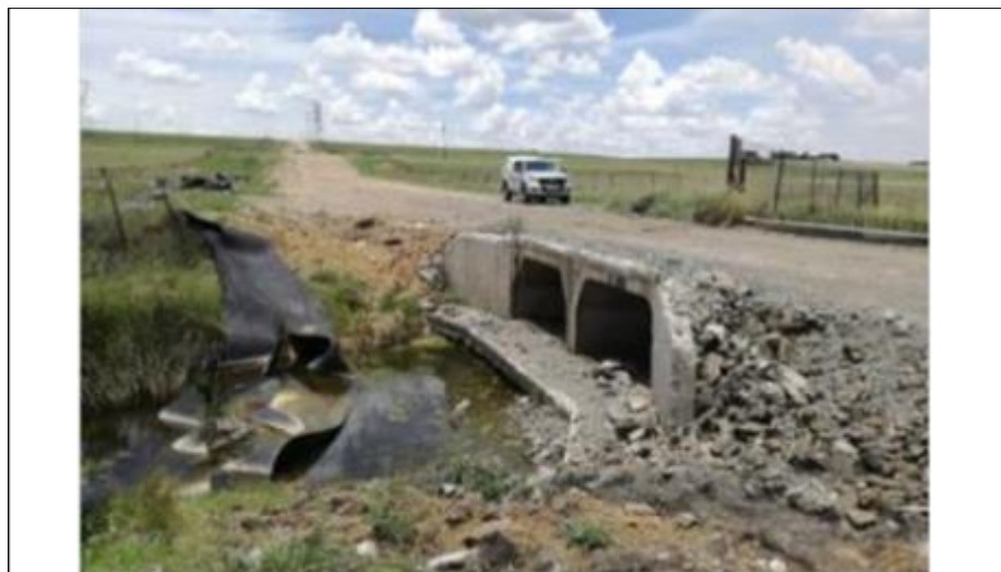
Photograph 5-2: Conveyor belt lying on the ground at a river crossing
