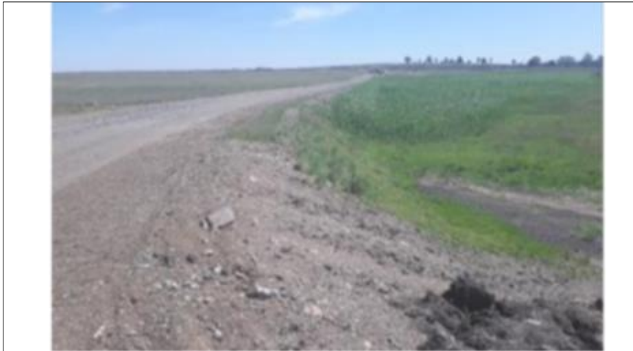
Photograph 5-5: Gravel road from Mynpad to the Twistdraai East Shaft area
