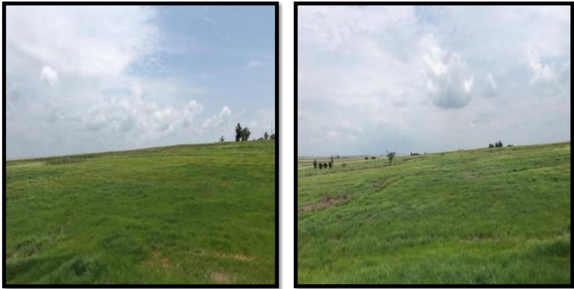
Figure 5-9: Rehabilitation of the two PCDs
