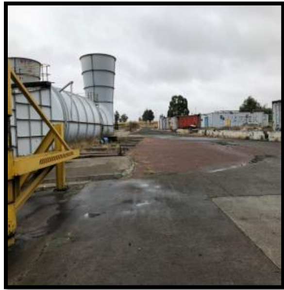
Figure 5-3: Twistdraai East Ventilation Shaft prior to decommissioning
