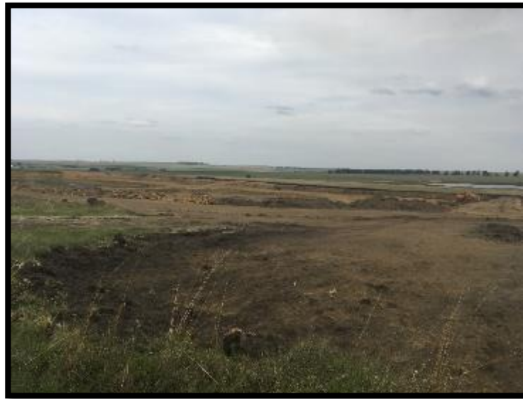
Figure 5-23: Quarry to be decommissioned and rehabilitated
