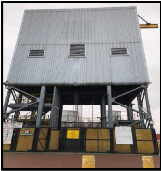
Figure 5-2: Twistdraai East Main Shaft prior to decommissioning
