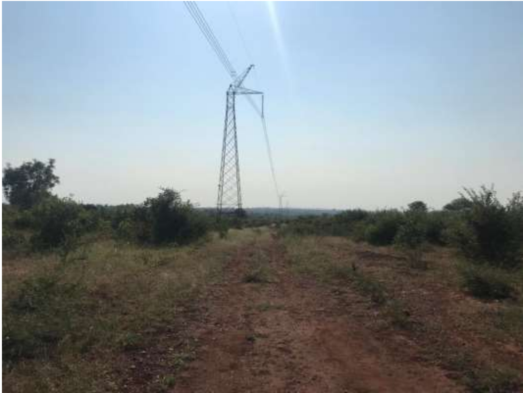
Figure 8: View of Eskom power line from Cahora bassa in Mozambique.
