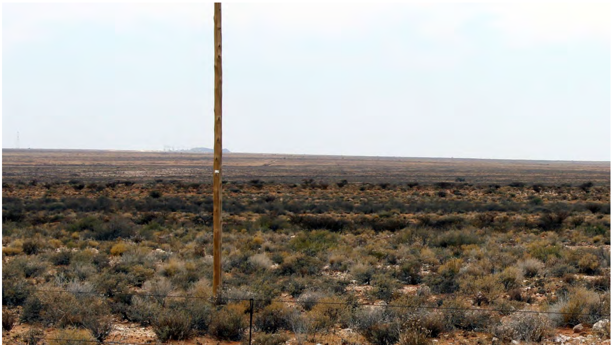
Figure 1-13 View from photo site SCA014 eastwards. The tower at Rugseer Siding is visible on the left and the new substation more towards the centre.
