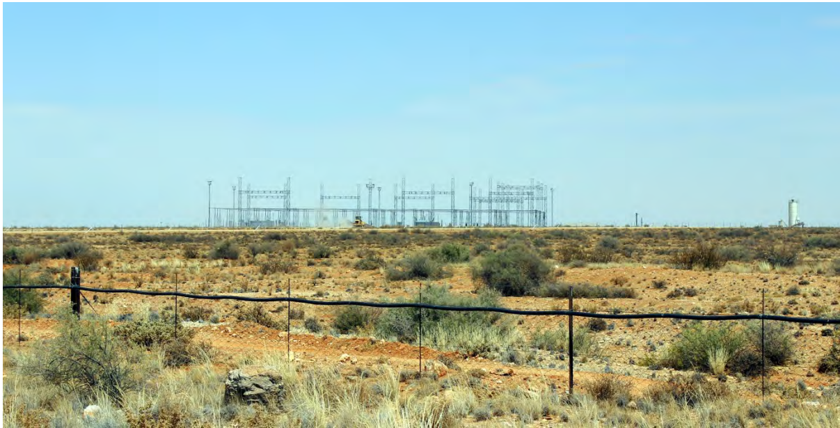
Figure 1-14 Eskom Nieuwehoop Substation currently under construction (Photo site SCA010)
