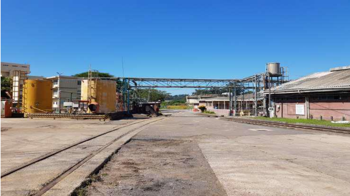
Figure 3 - rail infrastructure within the site premises (Source, Broll Information document, 2018).
