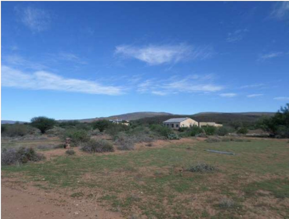
Figure 4: Portion 2 and 4 Rietfontein: Abandoned farm buildings
