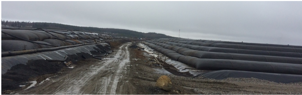
FIGURE 9-3: DE-WATERING BAGS USED FOR MINE WASTE
