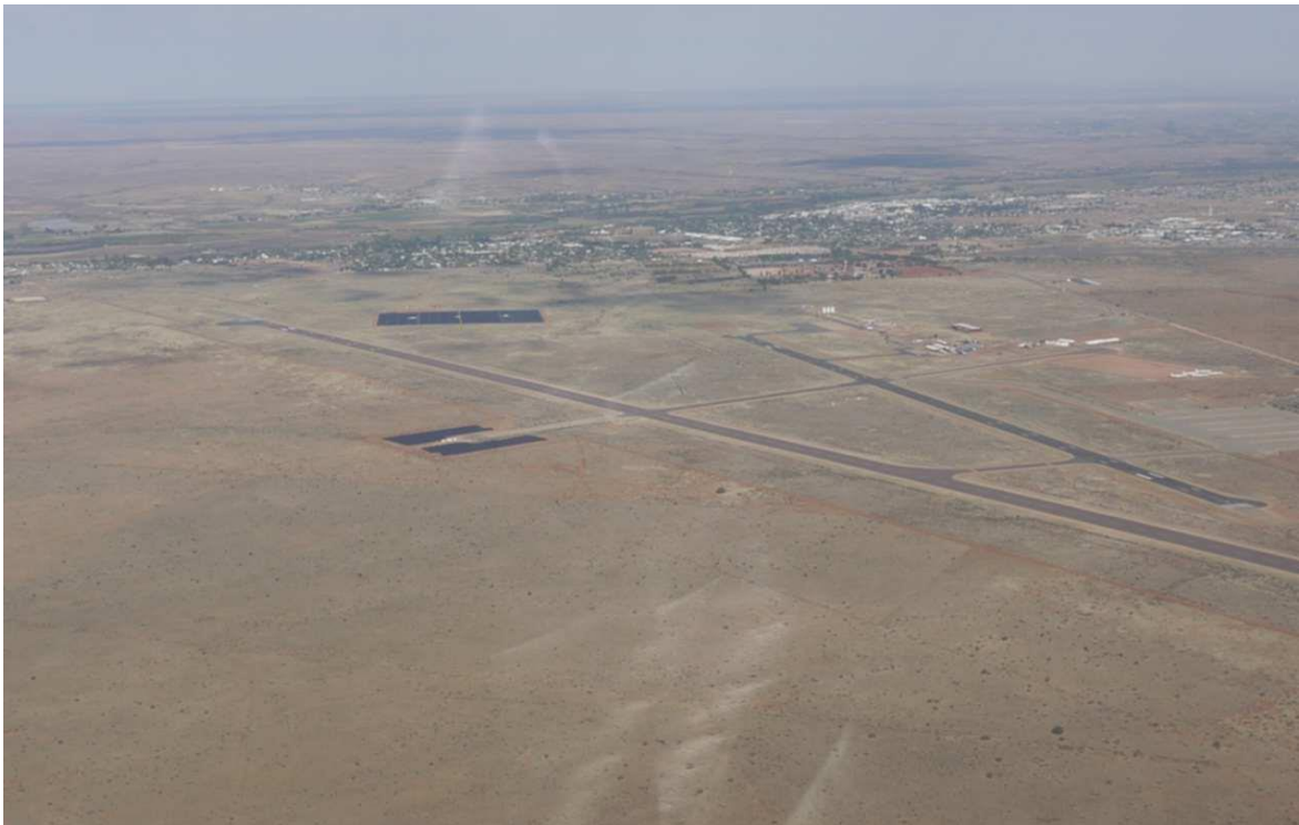
Plate 20 , Existing solar arrays at Upington Airport as seen from the air
