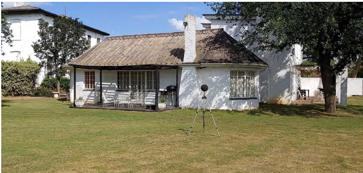
Photo B.2: Measurement location at WRLTSL02
