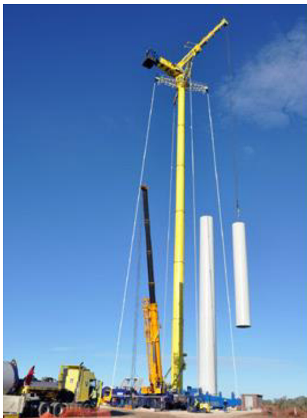
Figure 2.6: Example - Cranes at work
