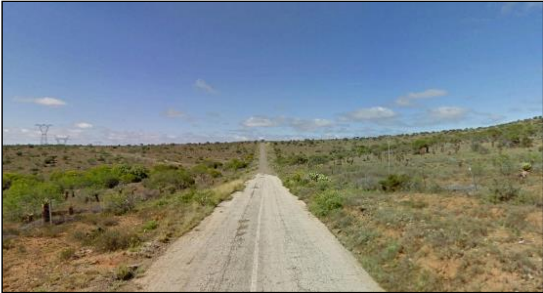
Figure 5: Access road from the N10 to the proposed Ripponn project site.
