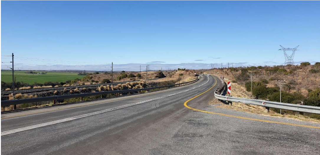
Figure 3-6: N10 Southbound at Access Point 2
