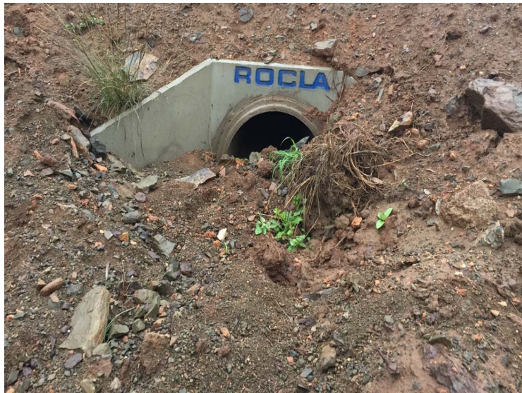
Figure 4 – Typical Stormwater crossing along DR02462
