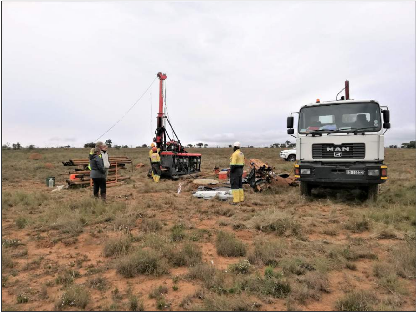
Plate 1: Rotary core drilling at borehole position E64
