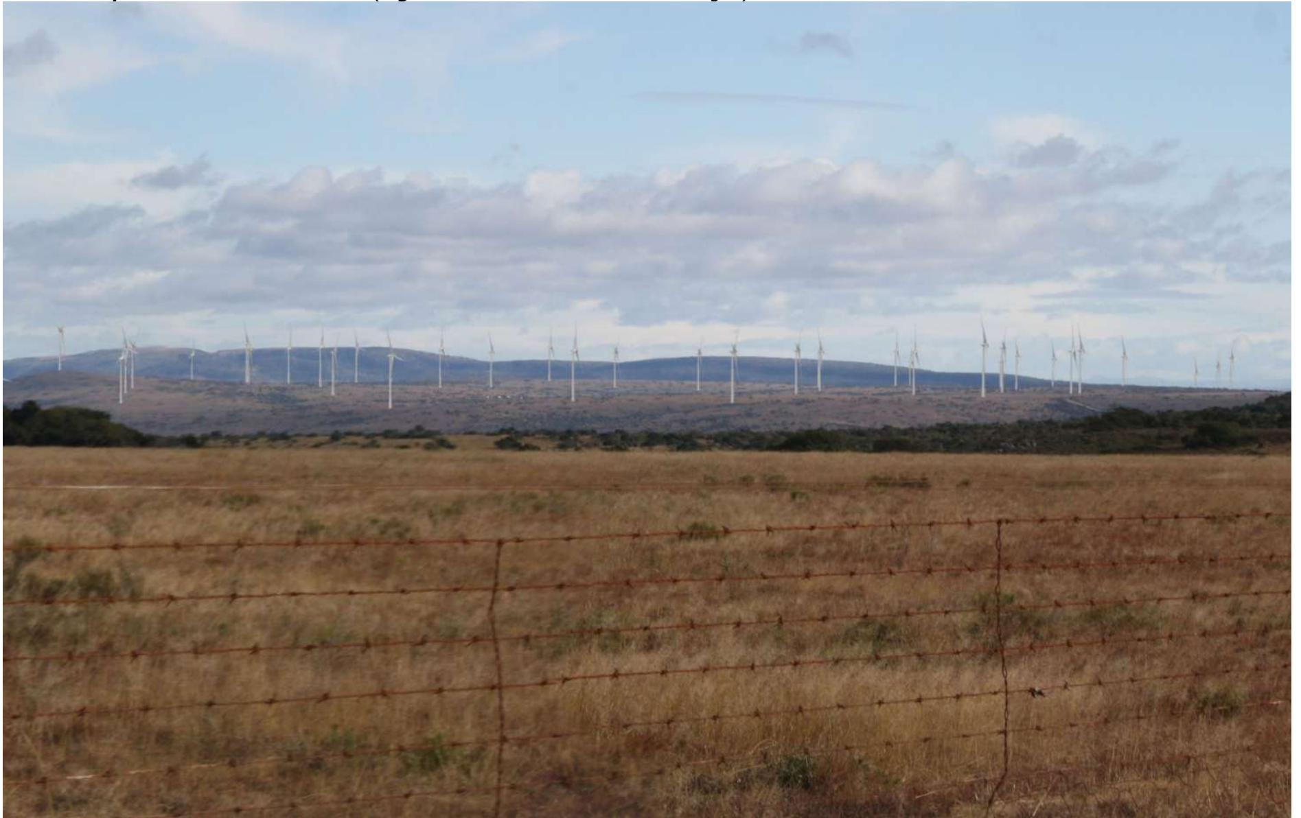
7.15. Viewpoint 5: after construction (Figure 26: Photo simulation 5 - enlarged).
