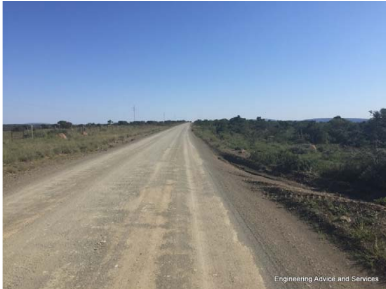
Figure 3 – Condition of Road MR00481
