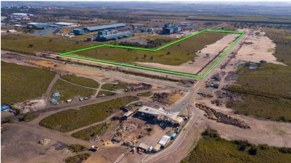
Figure 6.5: Photograph of the EIA footprint area and associated existing impacts
