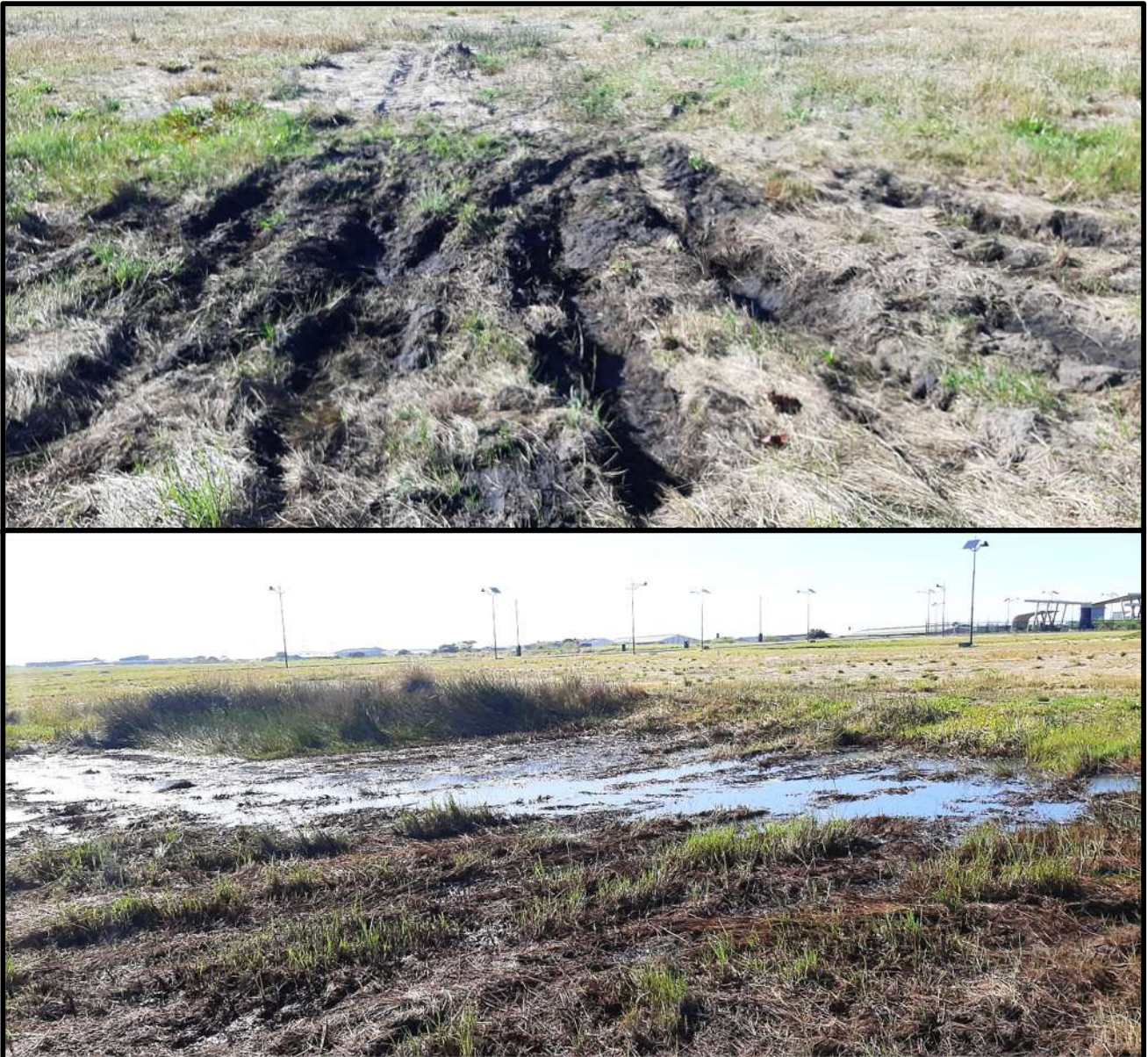
FIGURE 24: Site visit - 16/7/2020, after the infilling of the wetland on the project site.
