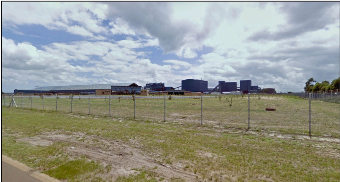
Figure 5: Existing steel works west of the proposed development site.
