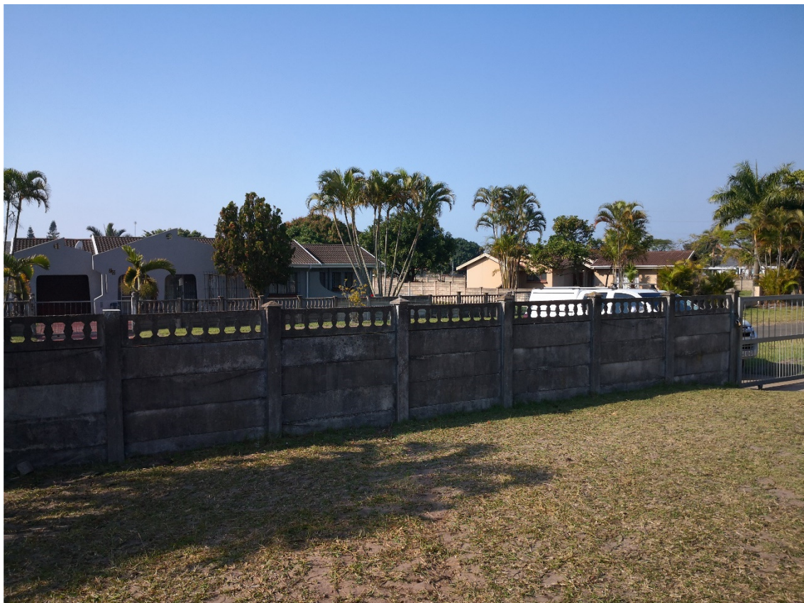
Photo B.1: Measurement location RBNSTSL01
