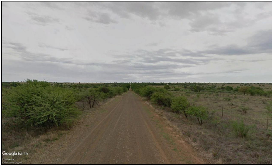
Photograph 5.5. Access road to the Vrede development area.
