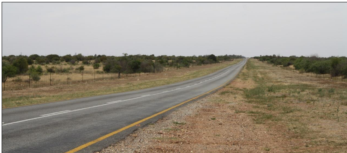
Figure 13: Thicket and bushland along the R505 – high VAC.
