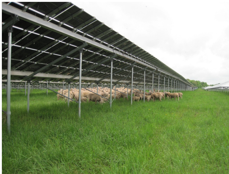
Figure 3: Solar plant in Toul-Rosières (France). Source: EDF Renewables France
