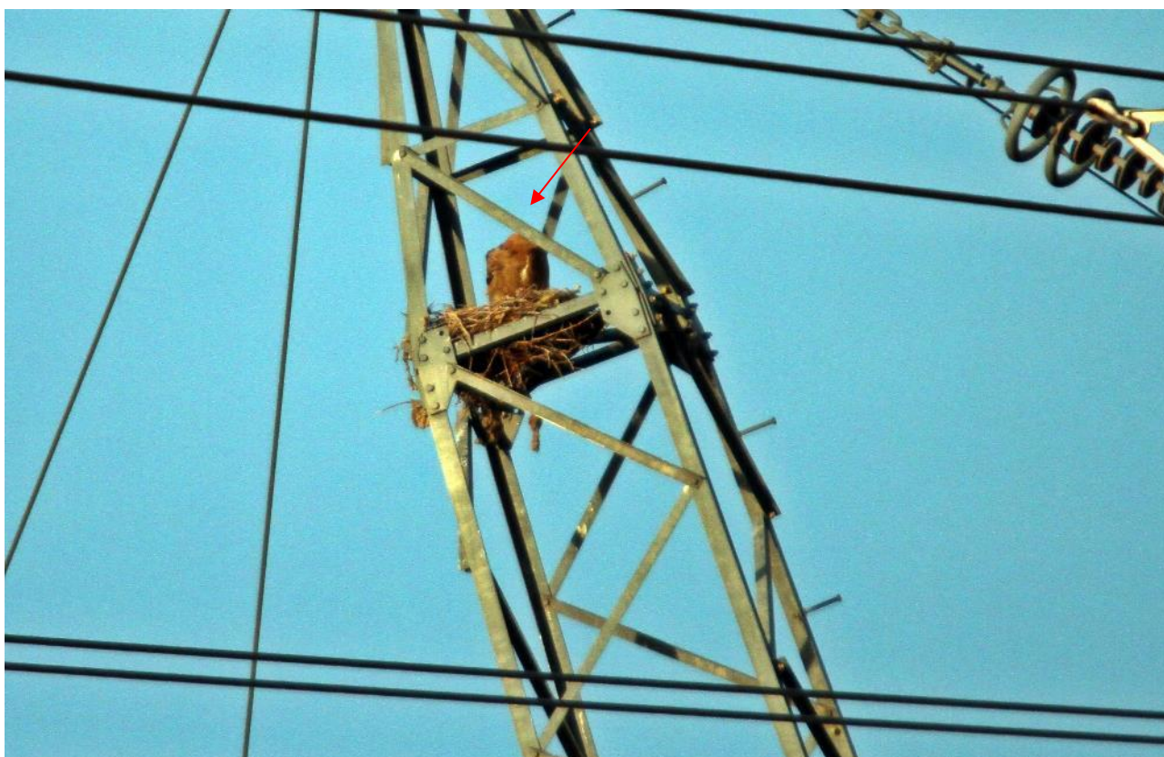
Figure 2: A Tawny Eagle nest (FPTE4) on the 1 Droërivier Hydra 400kV transmission line
