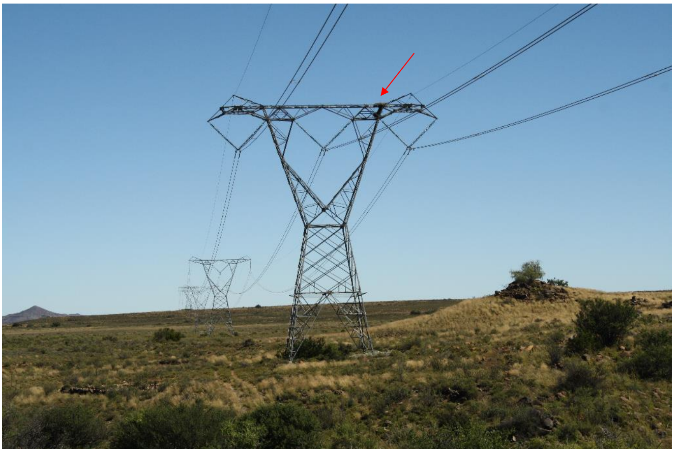
Figure 2: A Tawny Eagle nest (FPTE1) on the Droërvier Hydra 400kV transmission line
