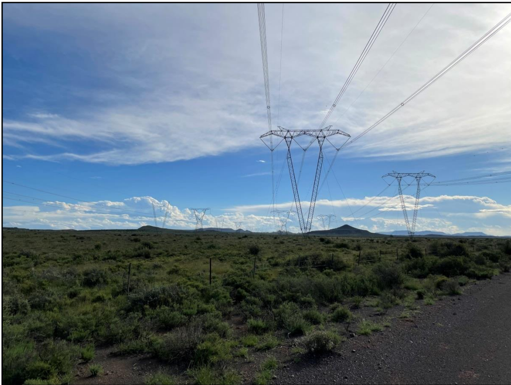
Figure 9: Existing power lines along the proposed alignment (looking to the south-west).
