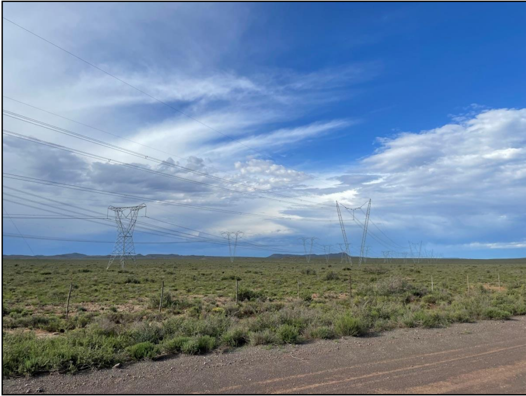
Figure 8: Existing power lines along the proposed alignment (looking to the north-east).
