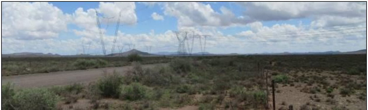
Photograph 3.5: Four (400 kV and 765 kV) Tx lines traversing the Hutchinson Road on Annexe Rondawel.
