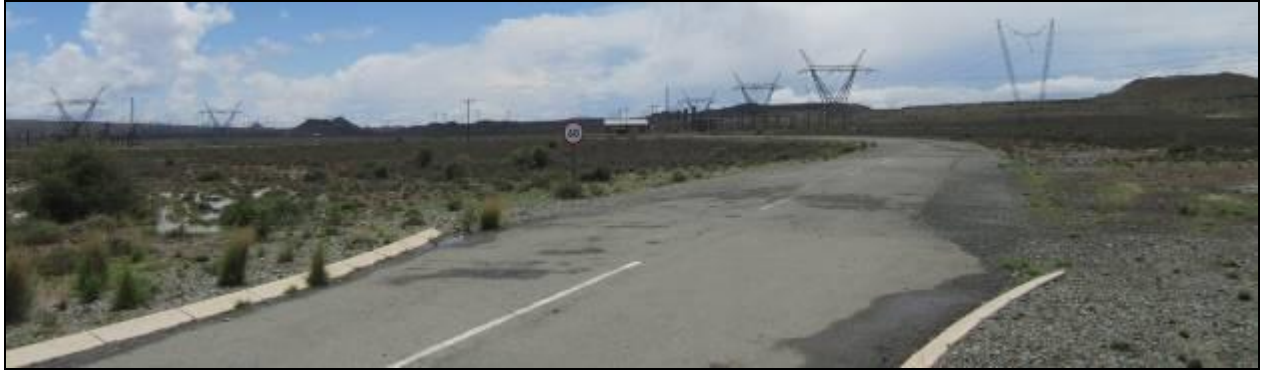
Photograph 3.4: Portion of Gamma on Schietkuil 3/1 into which the project would feed, located approximately 200 m north of the R63.
