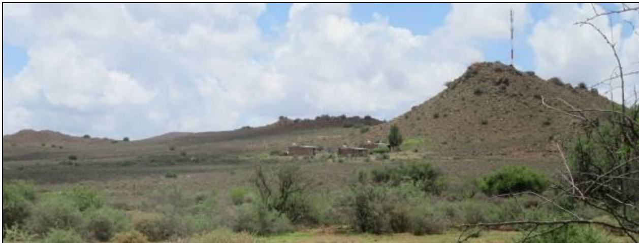
Photograph 3.10: Labourer's houses on Rondawel seen from the N1.
